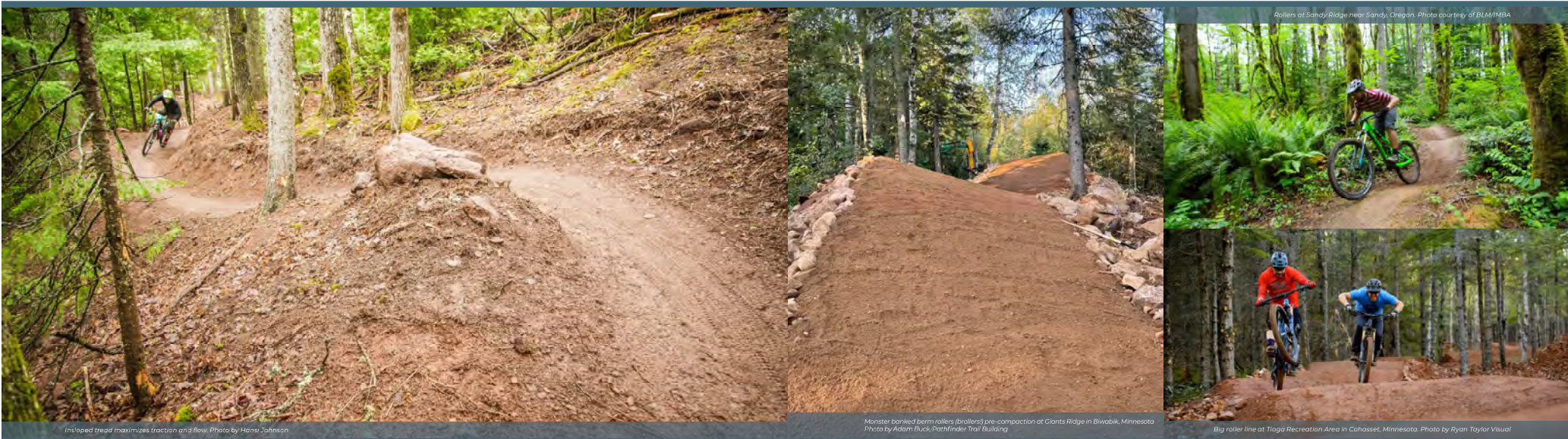
Insloped tread maximizes traction and flow. Photo by Hans Johnson
