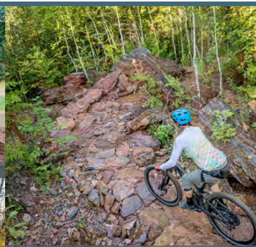
Constructed technical rock tread at Tioga Recreation Area in Cohasset, Minnesota. Photo by Chris Gilbert/Rock Solid
