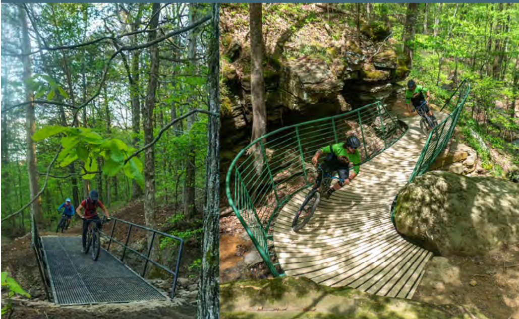
Prefabricated steel bridge at Devil's Den State Park in Winslow, Arkansas. Photo by Andy Fietstra/Rock Solid
