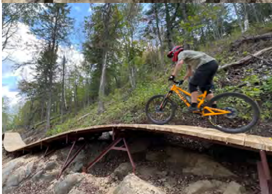
Custom steel-frame boardwalk with wooden decking at Giants Ridge in Blivak, Minnesota. Photos by Adam Buck/Pathfinder Trail Building
