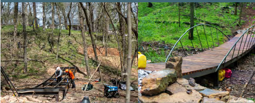
Steel-framed bridge with wooden decking at Headstart to Slaughter Pen in Bentonville, Arkansas. Photos by Eli Giesmann/Rock Solid
