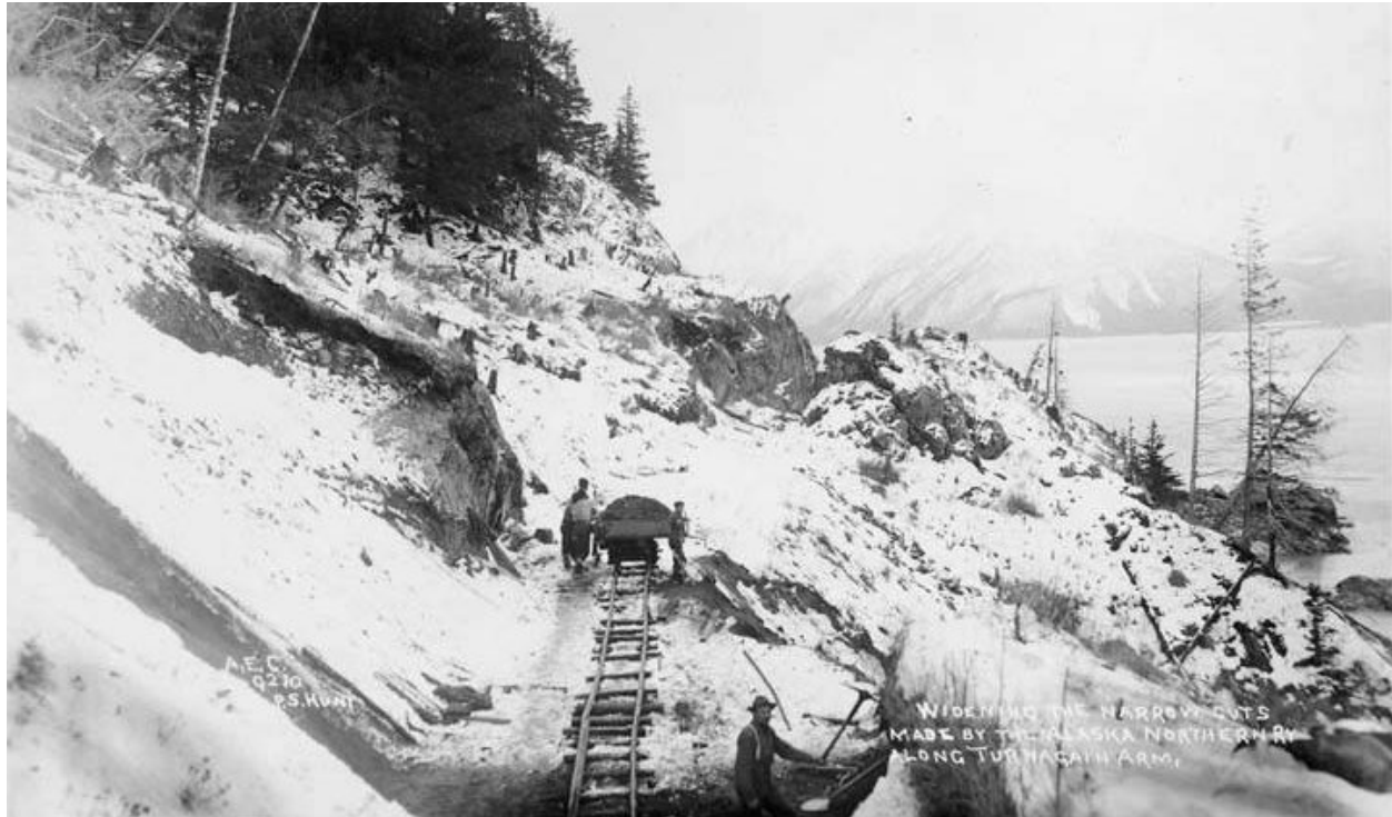
FIGURE 9: WIDENING THE CUTS MADE FOR THE RAILWAYS. UAF-2013-159-45
